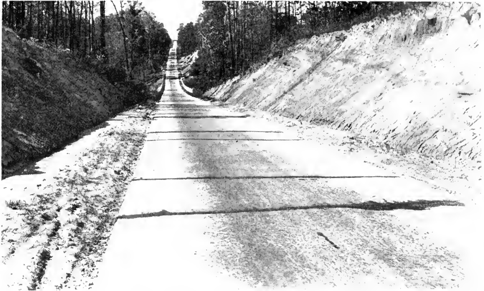
The superhighway of the Twenties was the Crain Highway—long, straight and the first on new location since the Eighteenth Century. It is now being rebuilt as one lane of newly-dualized U. S. 301. The original road cost $40,000 a mile.
